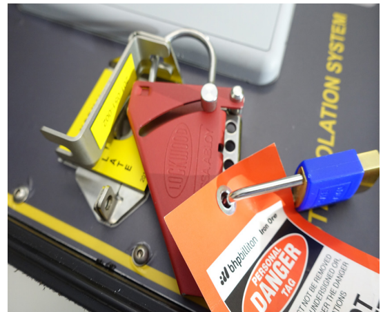
Isolator Lockout Switch (ILS)
